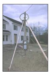
**Figure 5: Temporary Power Distribution Setups**
