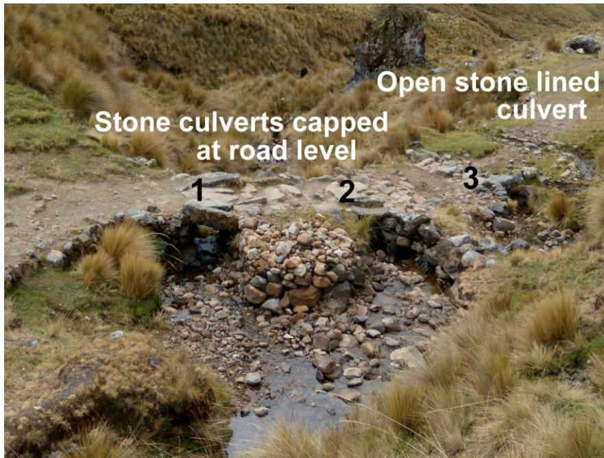
Figure 5: Inka Road Culvert north of Taulli
