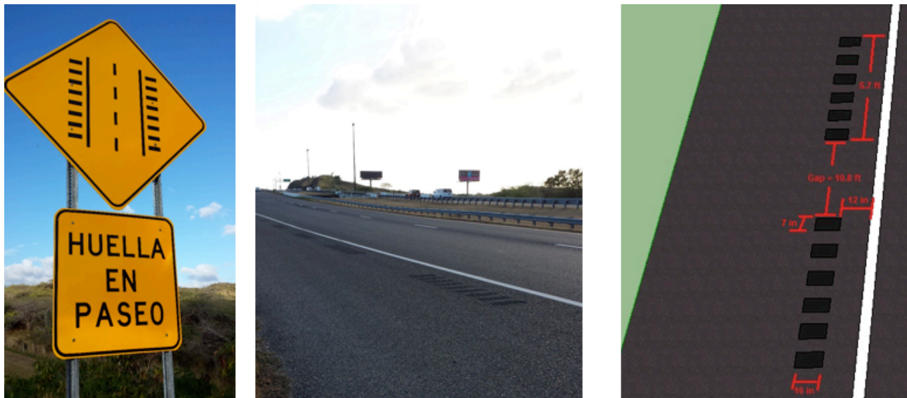
Figure 4: Rumble Strip Sign, Photo of the Rumble Strips on NHS PR-52 Freeway and Dimensions
