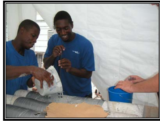
Figure 17: Repair 5 – Mix Pouring
