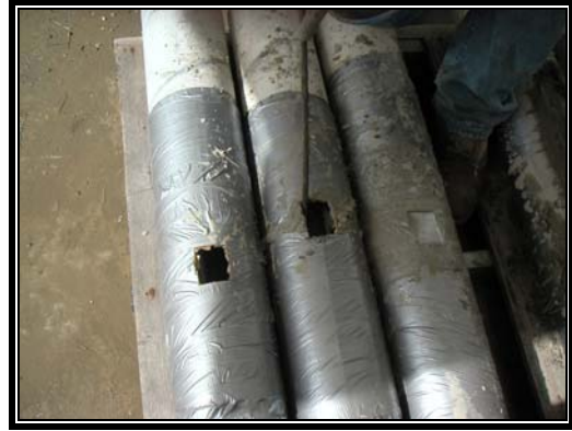
Figure 20: Repair 6 – Mix Pouring
