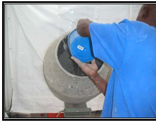
Figure 11: Repair 3 – Mix Preparation
