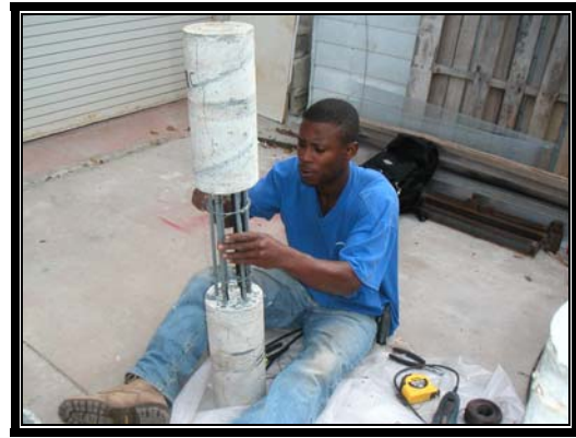
Figure 7: FRP Splicing of cylinders
