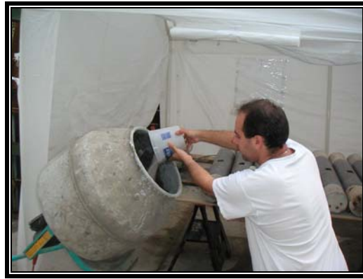
Figure 14. Repair 4 – Mix Preparation
