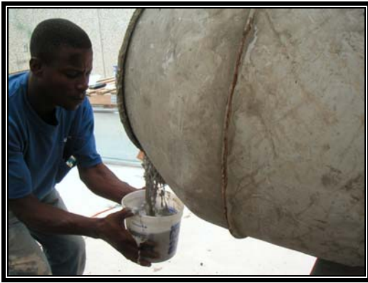
Figure 16: Repair 5 Mix Preparation
