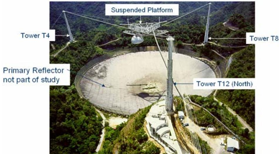
**Figure 1: Overall view of the Arecibo Observatory (courtesy of NAIC)**
