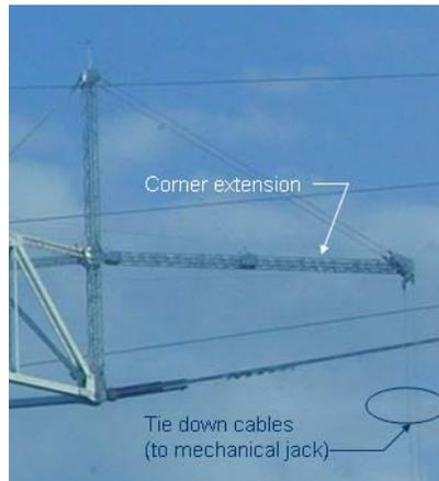
**Figure 6: Tiedown cables and platform attachment points (courtesy of NAIC)**
