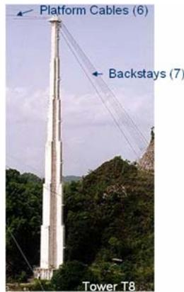
**Figure 3: Tower T8, the tallest (365 ft) of the three towers. (courtesy of NAIC)**
