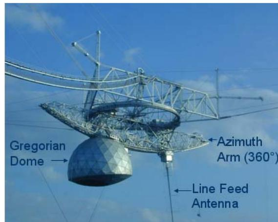
**Figure 2: Suspended platform and its main components (courtesy of NAIC)**
