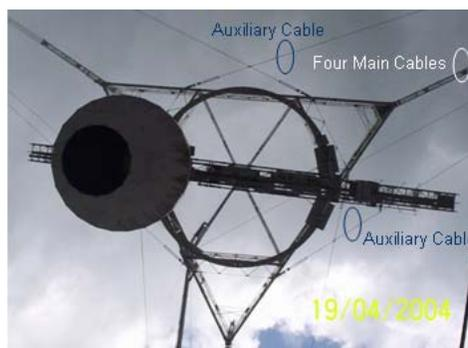
**Figure 5. Attachment points of cables to platform. T4 cables highlighted. (photo by author)**
