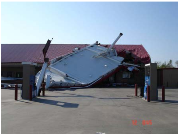
Figure 2a. Exxon Gas Station, Road 365 and Labelle Road, Hillerbrandt, TX (Photograph taken on October 12).
