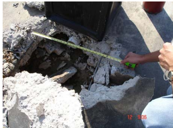
Figure 2b. Exxon Gas Station, Hillerbrandt, TX (Photograph taken on October 12).
