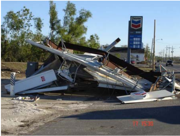
Figure 8a. Chevron gas station in Meraux, LA. (Photograph taken on November 17).
