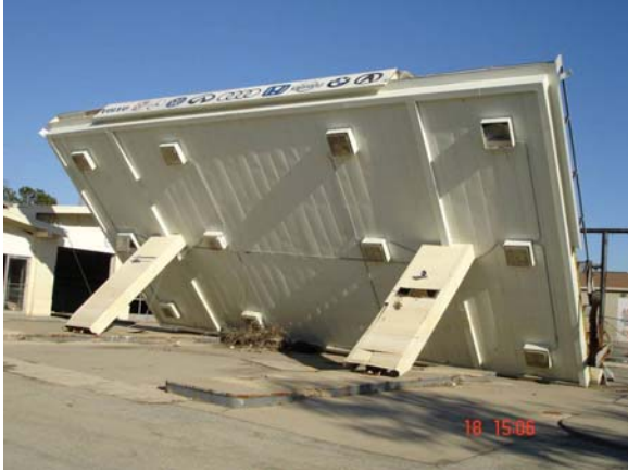
Figure 5a. Road 39, Chalmette, LA. The connection between column and roof was effective. (Photograph taken on November 18).
