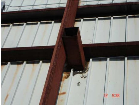
Figure 3c. Exxon Gas Station, Hillerbrandt, TX. There was effective frame action. (Photograph taken on October 12).
