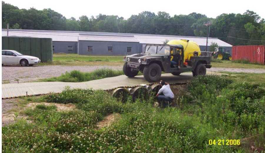
Figure 12: HHMMV Defeats the 9ft Gap
