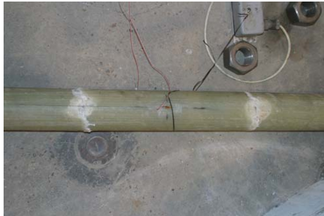
Figure 4: Area of Compression Failure in 3in Pipes
