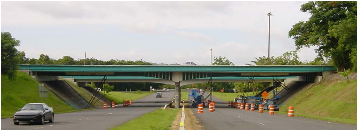
Figure 1 Bridge 2028 After Rehabilitation with CFRP
