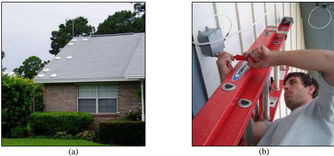
Figure 6: (a) sensors mounted on roof (b) sensor mounted on wall
