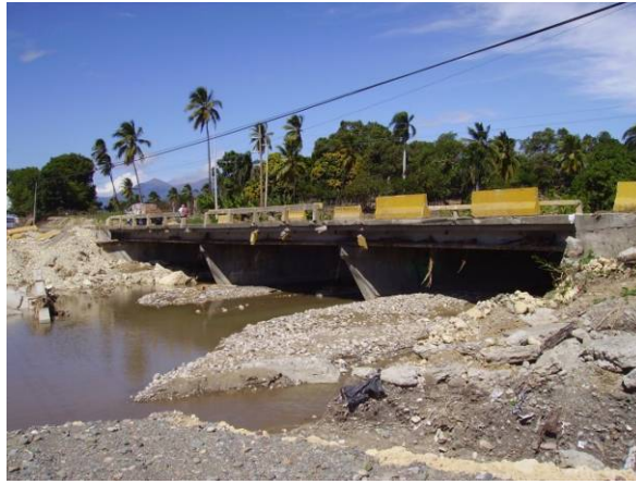
Figure 6: Paya River Bridge
