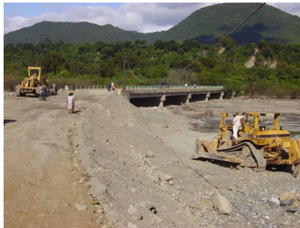
Figure 5: Reconstruction of San José de Ocoa Bridge
