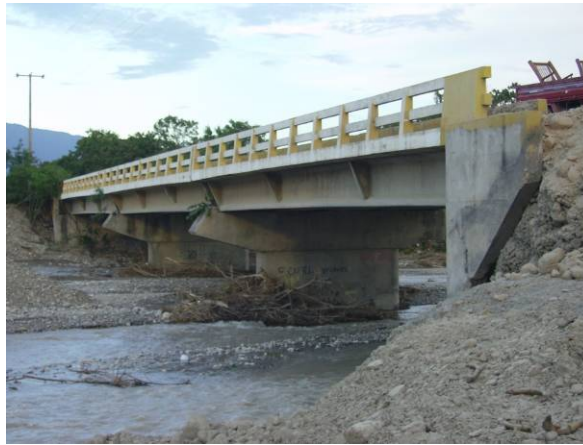
Figure 4: Los Jovillos Bridge
