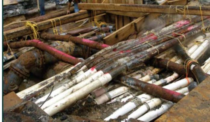
**Fig. 1: Actual subsurface interference picture in NYC**
