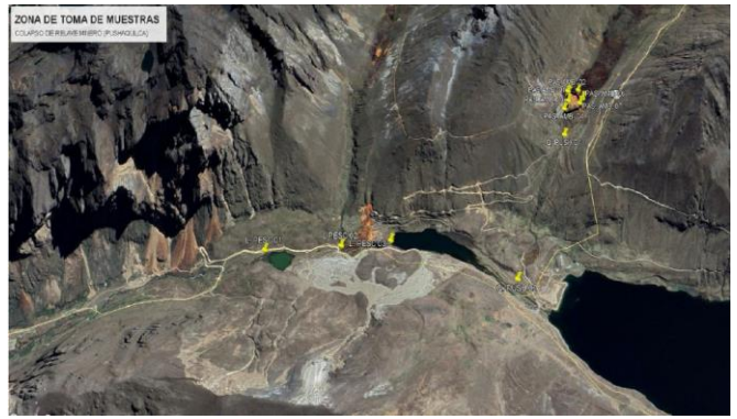
Fig. 3 Satellite image of the monitoring point
